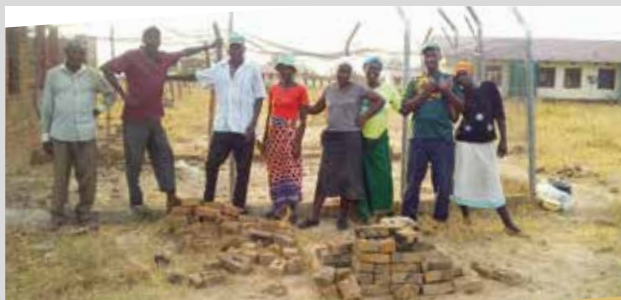
Members starting work building the new Carpentry Workshop
